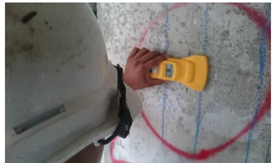
COVER METTER TO SCAN STEEL BAR POSITION
