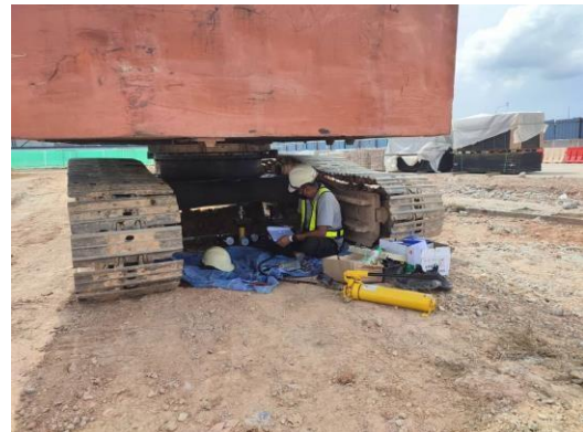
PLATE BEARING TEST
